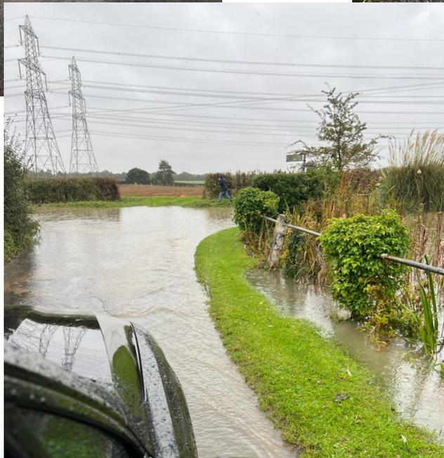
Presmere Pond couldn't cope with the amount of rainfall and taking water from nearby drainage ditches. It overflowed into adjacent roads. The flood was finally released when grips were opened up and the water flowed into the field ditch.
